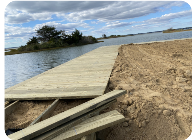
BOARDWALK AND BULKHEAD REPLACEMENT – NPS, MD
